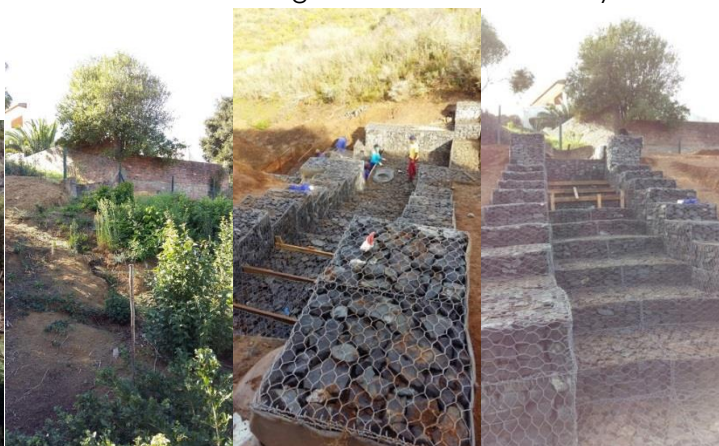
Figure 32: After photos - View down and up slope of the TNR gabion project.
